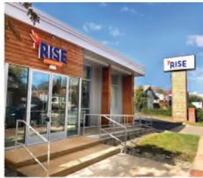
EXTERIOR OF RISE SILVER SPRING Silver Spring, Maryland
